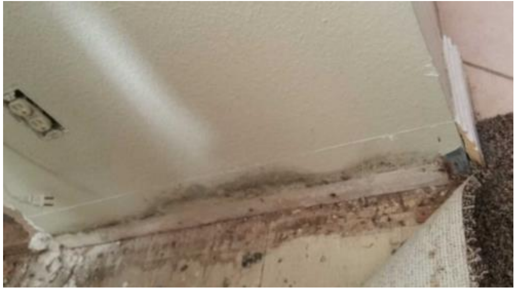
9 Level 2/Master Bedroom - 14-CID 03-06-Ken (5) Date Taken: 3/6/2017
