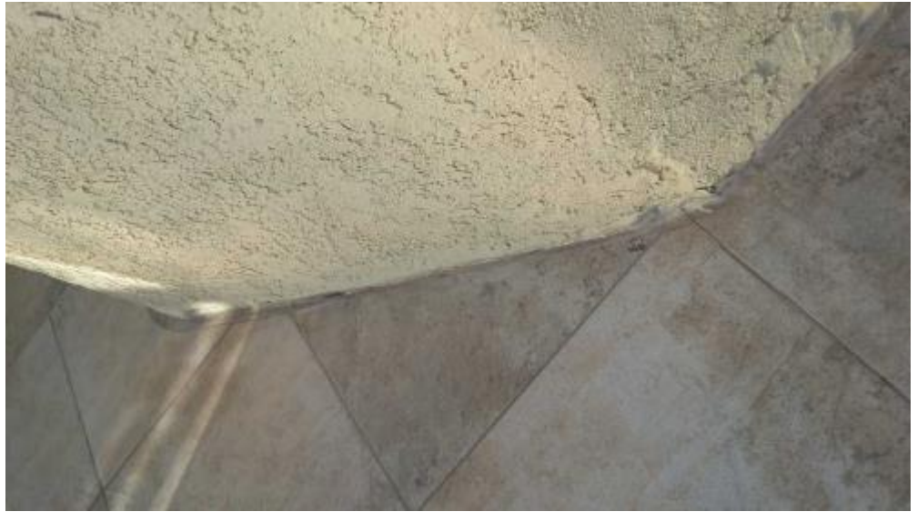
11 Level 2/Master Bedroom - 16-CID 03-06-Ken (14) Date Taken: 3/6/2017
