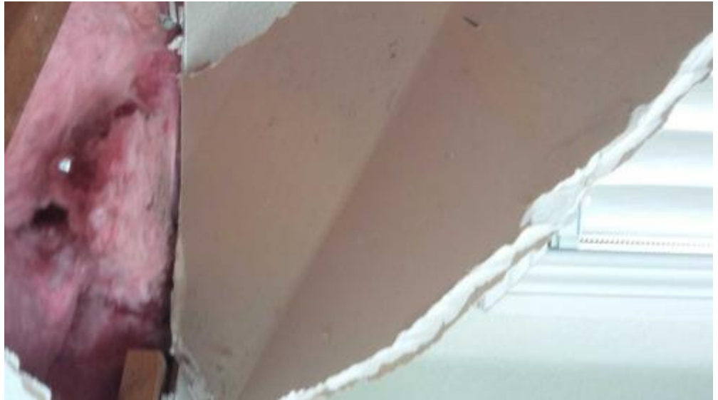
10 Level 2/Master Bedroom - 15-CID 03-06-Ken (6) Date Taken: 3/6/2017
