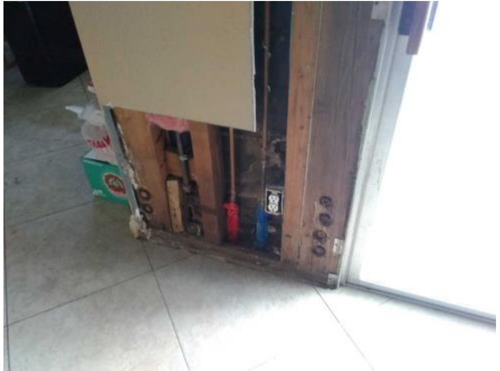
3 Main Level/Living Room - 10-P_ 20170213_163458 Date Taken: 2/13/2017
