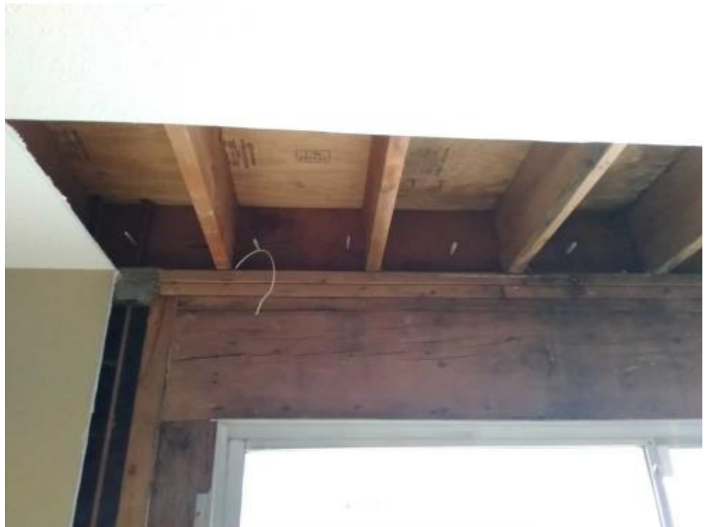
2 Main Level/Living Room - 9-P_ 20170213_163447 Date Taken: 2/13/2017
